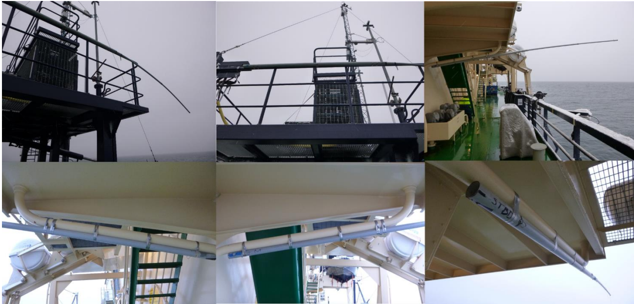
Figure 5. Detail of outrigger positions and means of attachment to hull features.
